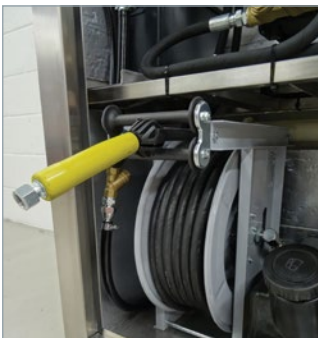
RETRACTABLE POWDER COATED STEEL HOSE REEL
